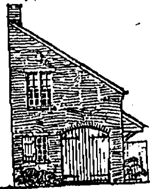
VIEW FROM NARROW COURT - EAST SIDE
